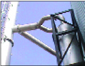
Common exhaust piping (not recommended)
